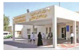
Psychiatric Hospital: Supply, testing & commissioning of Honeywell Trend BMS.
