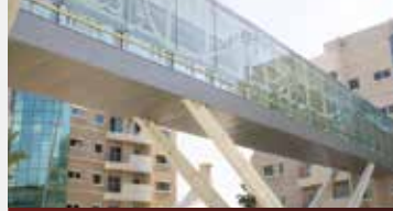
Construction of a Connecting Bridge.
