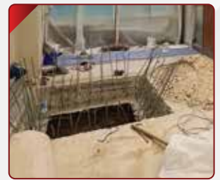
Facility Extension & Renovation
