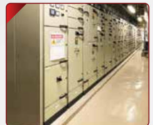
BMS & Access Control
