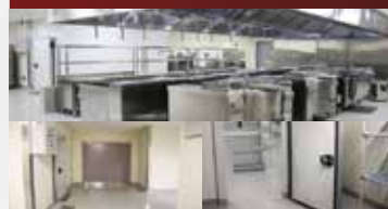
Fit-Out Works- Kitchen Modifications
